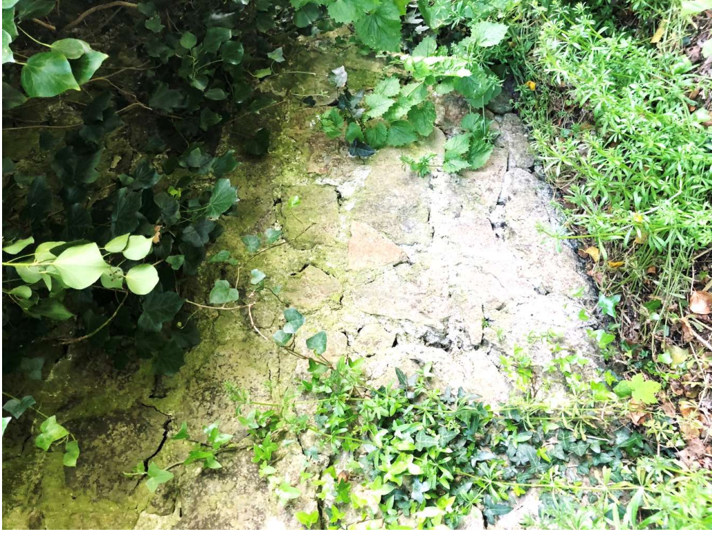
7. Detail view of the historic demesne wall to Howth Castle
