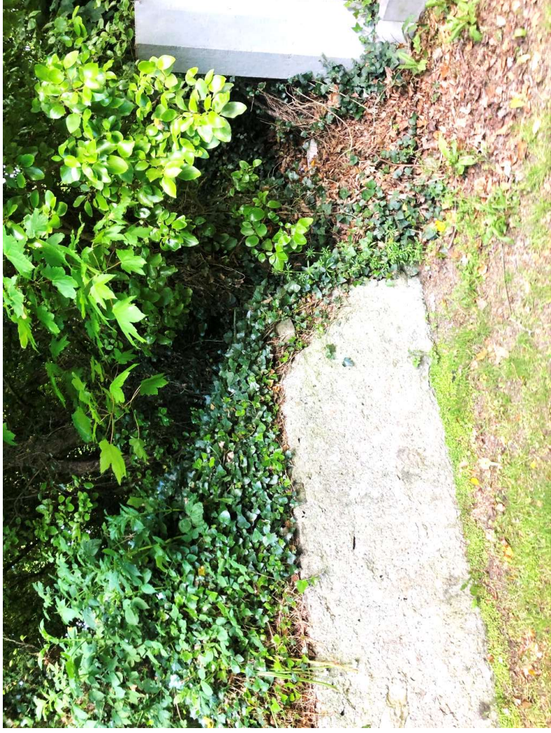
20. View of the junction between the historic boundary wall and the Entrance Gates to Howth Castle
