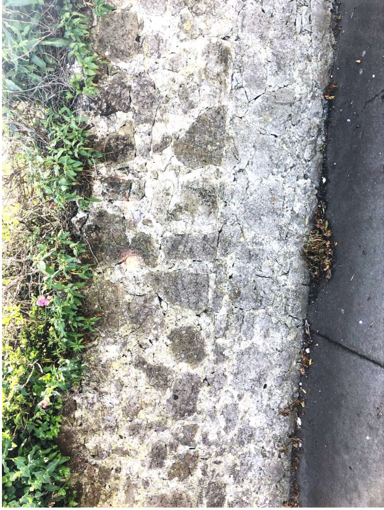
41. View of the historic demesne wall to the west along Howth Road
