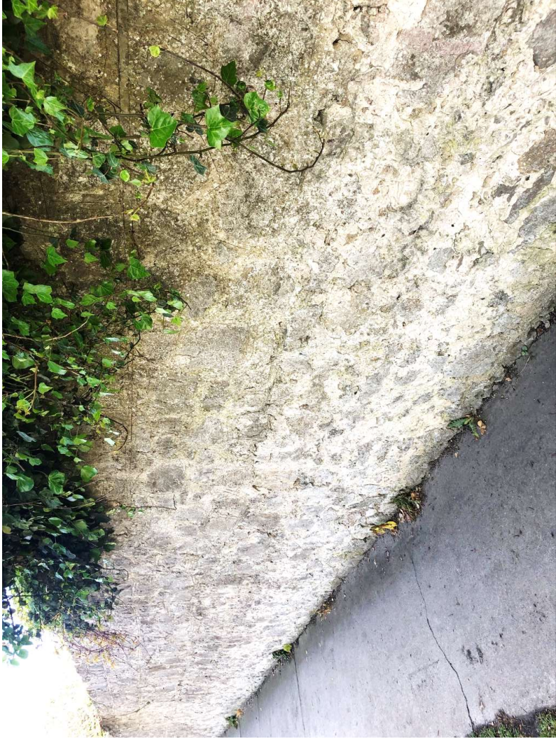
49. Detail view of the boundary wall to the northern boundary of the subject site
