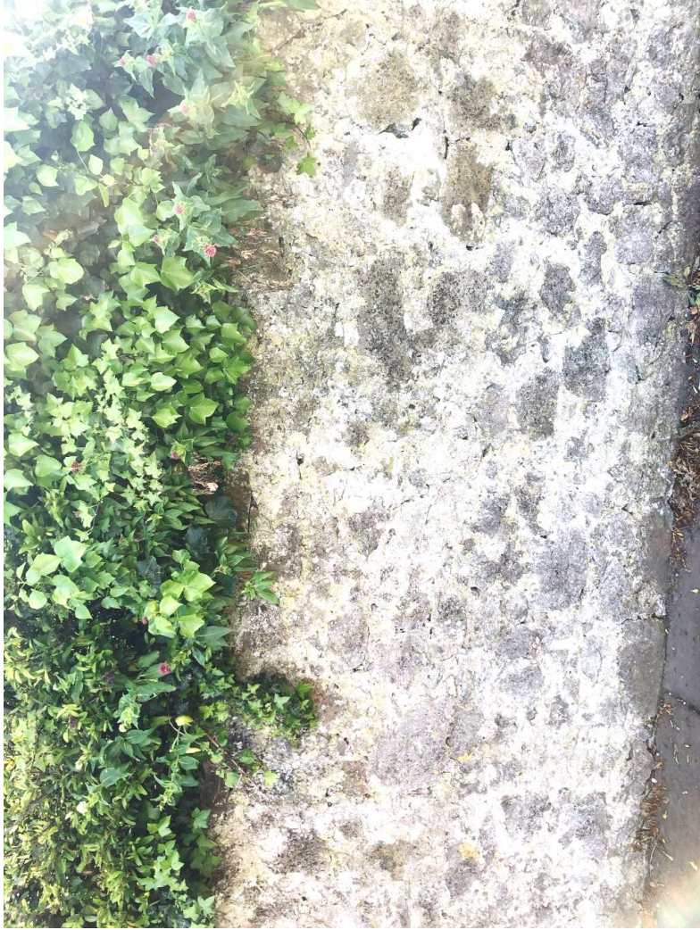
42. View of the historic demesne wall to the west along Howth Road
