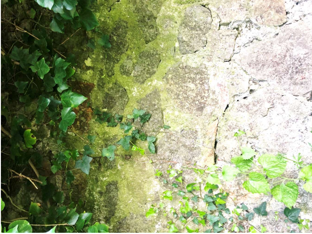
6. Detail view of the historic demesne wall to Howth Castle
