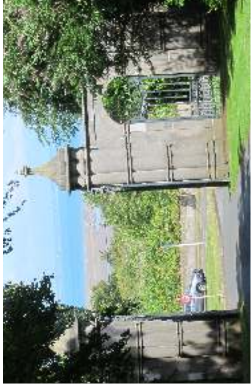
View from inside the main entrance gates across Howth Road to the Techcrete site, with sea in the background
