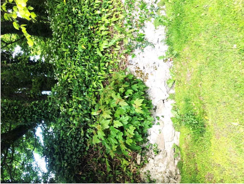
13. Detail view of the historic demesne wall to Howth Castle
