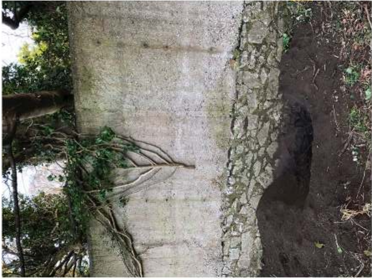
The wall along the boundary between the site and the castle within the entrance gates is mainly of modern poured concrete construction supported by remnants of the original wall at base.
