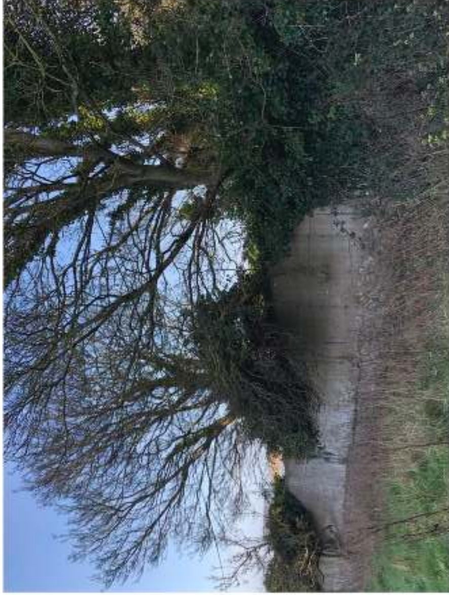
The wall along the boundary between the site and the castle within the entrance gates is mainly of modern poured concrete construction supported by remnants of the original wall at base.
