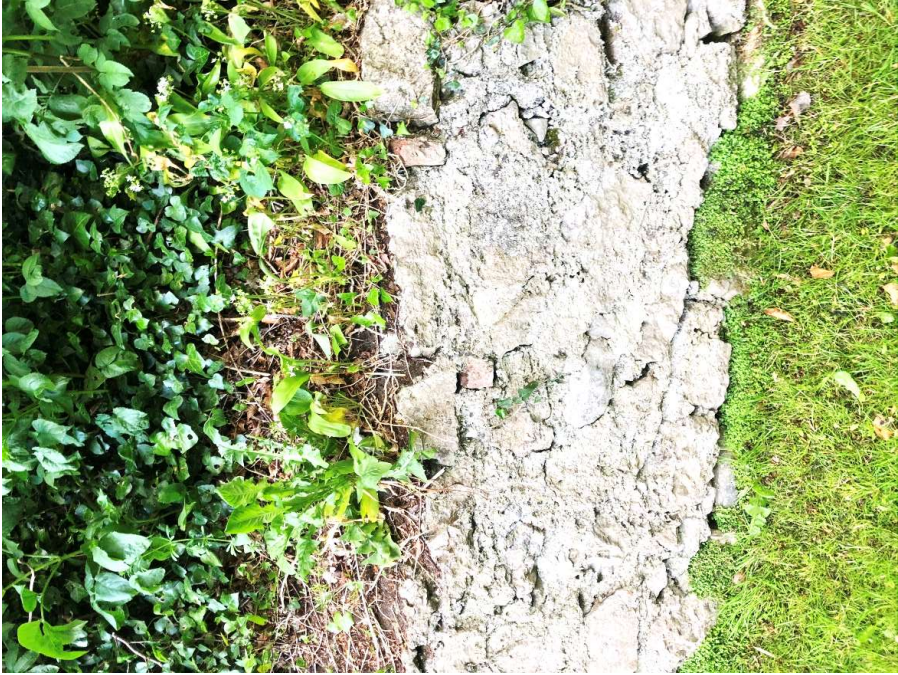
17. Detail view of the historic boundary wall
