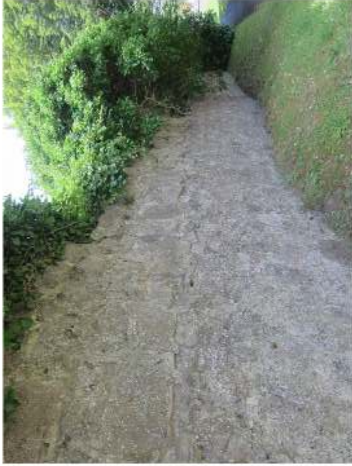
The demesne wall, Howth Road, the upper section of which has been rebuilt.
