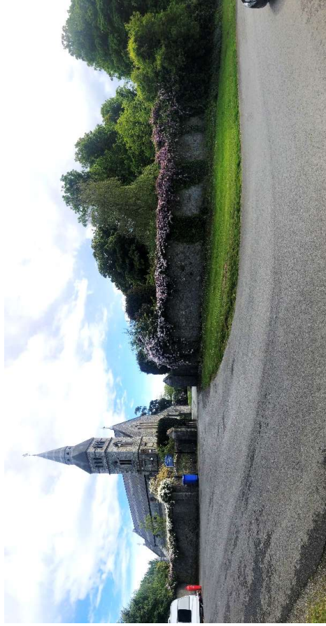
4. Panoramic view of the boundary wall to St. Mary's Church
